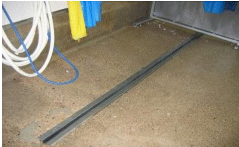
Figure 3.2: Slaughtering facility with a slanting floor and slot drainage
